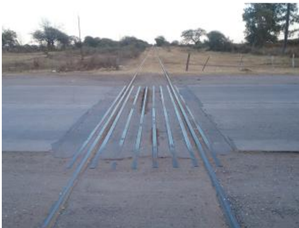
Figure 7. View of the level crossing, ascending direction of RP 3
